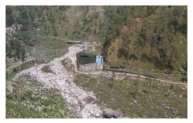
This small Hydroelectric Project is a run-of-river project on Baner Khad stream in district Kangra, Himachal Pradesh. The project has a generation capacity of 6.0 MW of power by utilizing the
