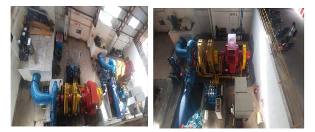
The project activity involves 2 numbers hydro turbine generators of Francis Horizontal axis type (3000 kW each) with internal electrical lines connecting the project activity with local evacuation facility.
